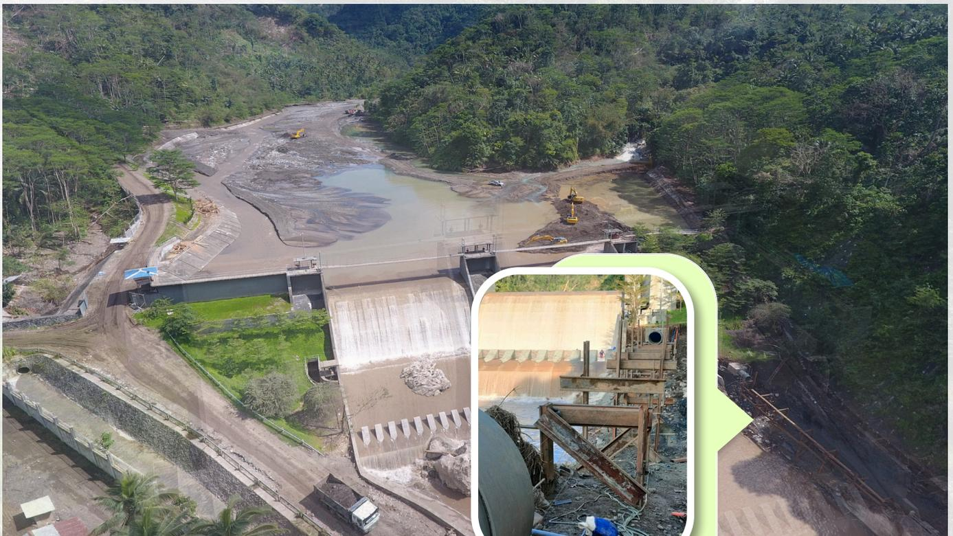
Conveyance pipe from impounding dam to the treatment facility was also damaged.
